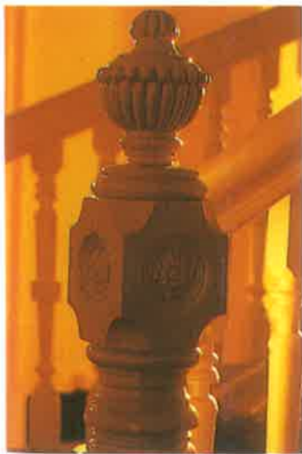
領事官邸之欄杆柱 充滿了精美雕飾。 Finely carved staircase newel post, consular residence.
